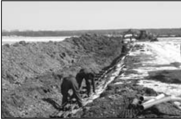
Personnel working on the Comms Loop on the north side of 8 Wing/CFB Trenton.
